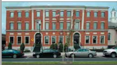
YMCA North Branch - 19 East Avenue - Lockport
